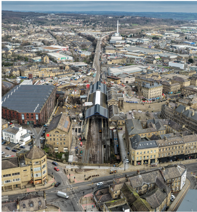
Railway improvement work is underway
